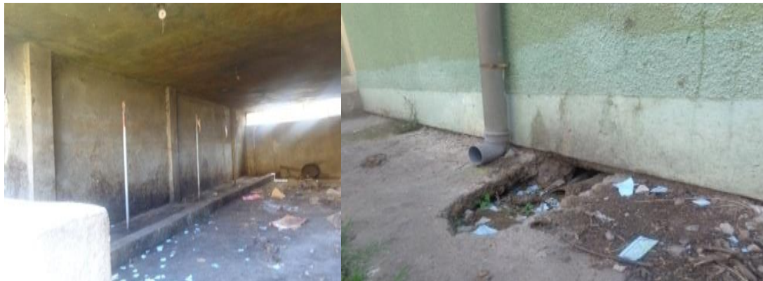
Figure 9: Unclean Slaughter House and Improper Disposal of Liquid Waste from the Slaughter House through a Hole
