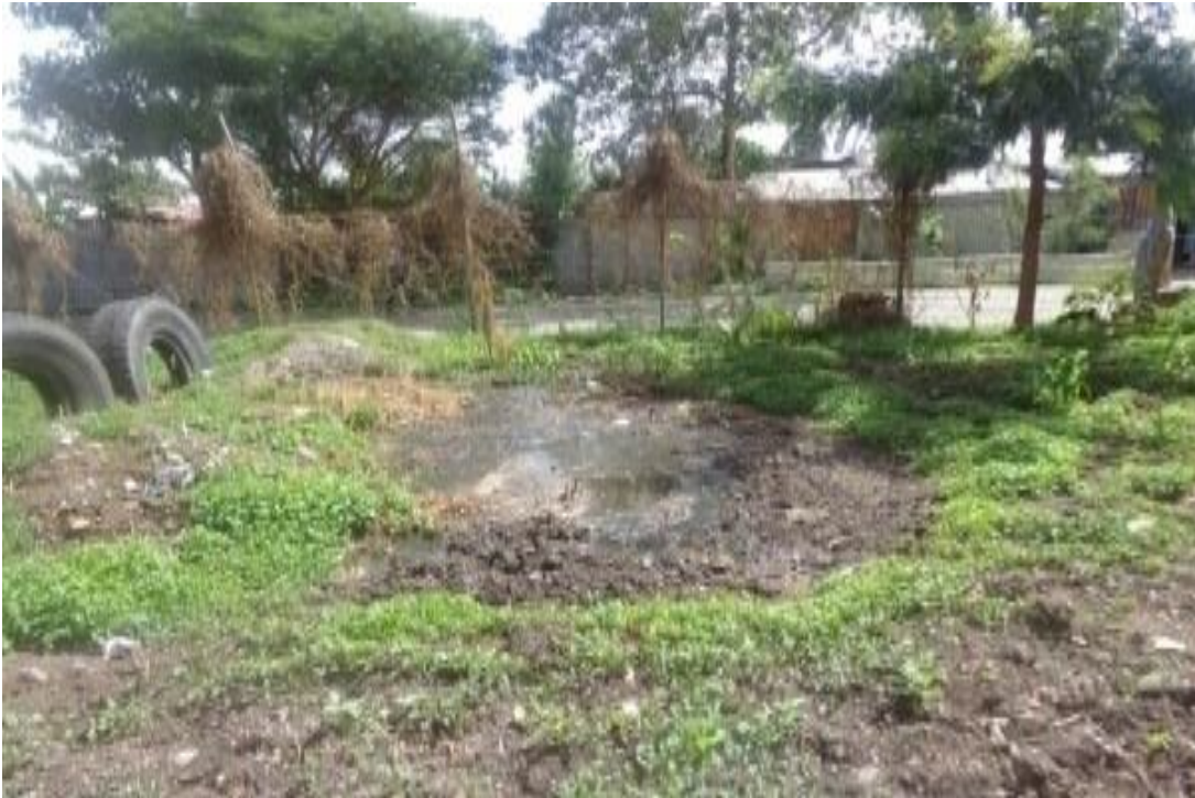
Figure - 8: Accumulated Liquid Waste from Liking Septic tank
