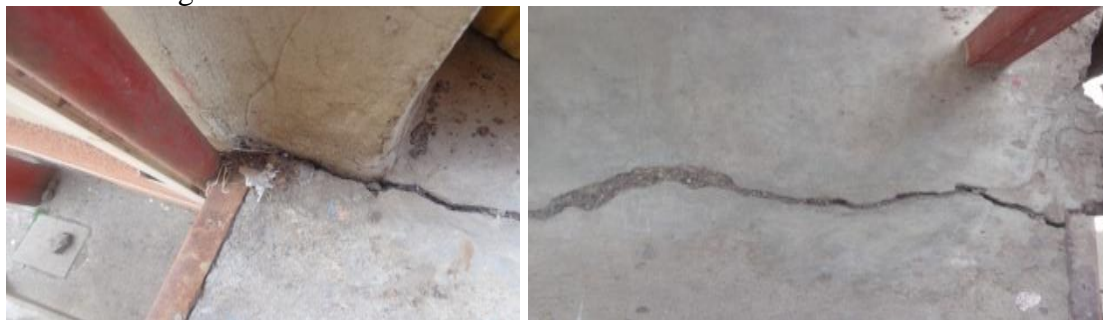
Figure - 4: Cracks on Stair Case Joint between two Adjacent Condominium Blocks
